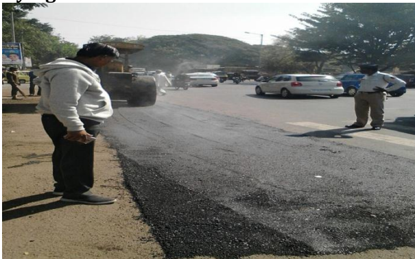
Fig-4: Bituminous mix lying on site
