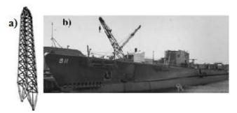
**Fig -2:** a) "Single lattice construction" sheerleg crane boom b) SS-192 crane construction as an example
