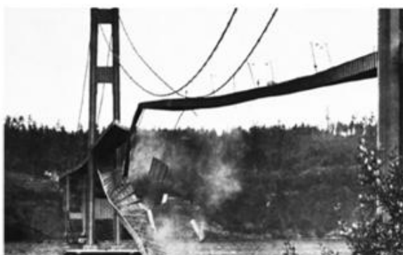
Figure 3. Tacoma Narrows Bridge an example of structure failure due to vibrations.
