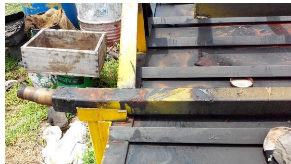
Fig2. bending problem of square axel trolley
