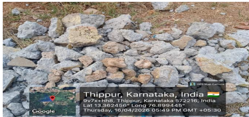
Fig 1.1 Demolished Concrete Wastes
