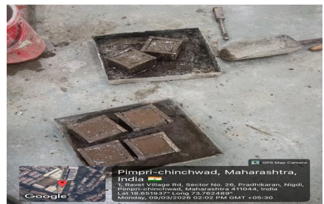
Fig 4.1.2 Curing of Concrete Cube Specimens
