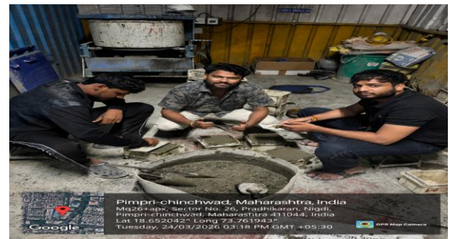
Fig 4.1.1 showing cube casting of Concrete specimens at site
