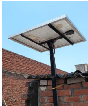
Fig. 7 , Fig -8: Rotatable Solar Panel Mounting Structure with Manual East–West Tracking Mechanism
