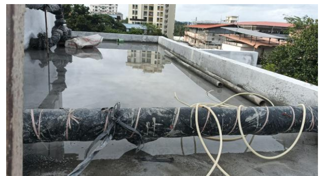
Fig -3: Commercial building for Mr. Justin Alookaran, Thrissur
