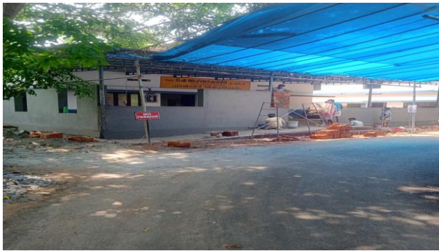
Fig -4: Renovation works at Family Health Centre, Puzhakkattiri, Malappuram
