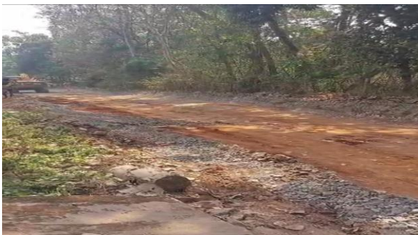
Fig -7: Demolition & re-construction of Road at Valakavu to Puthur (BMBC), Thrissur
