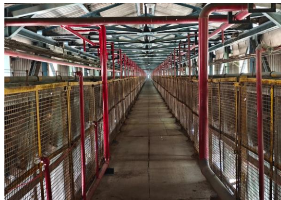
Figure 4: Additional gallery view supporting route scale and maintainability discussion
