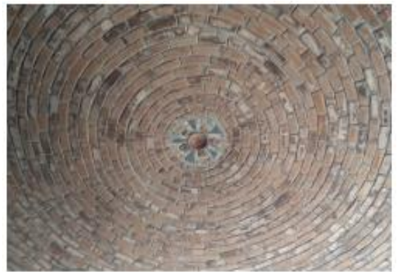
Fig -2: Rohtak Domes (Interior)
