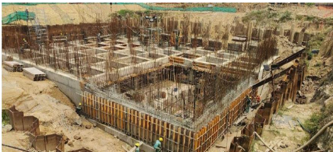
Figure 5-3 First lift wall casting - CRWS
