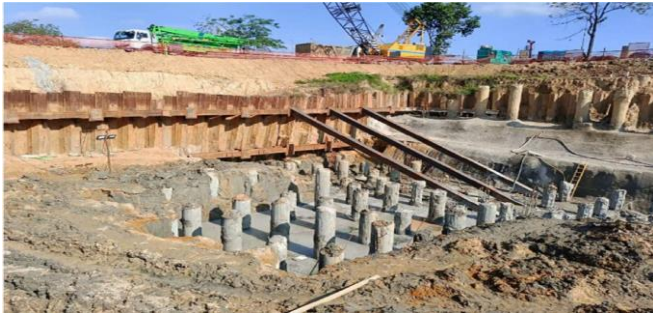
Figure 5-2 First Level Raker Support
