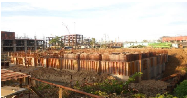
Figure 5-4 Final wall and slab - CRWS
