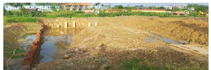
Figure 5-1 Sheet Pile Installation and 1st Level Excavation
