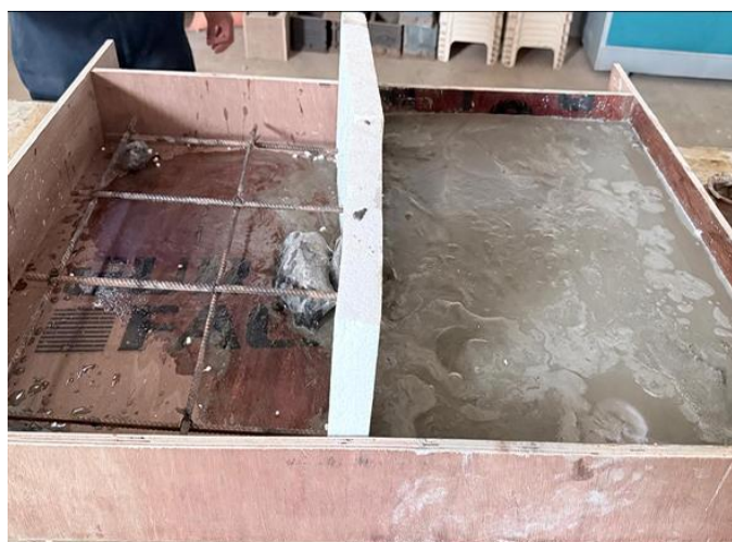
Fig -3: Curing of a filler slab
