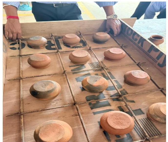
Fig -1: Slab Formwork
