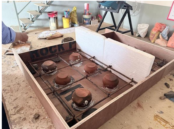
Fig -2: Arrangement Details for Filler Slabs
