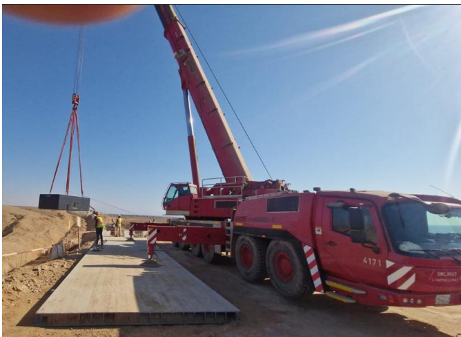
Fig.5: Wall Precast segment erection
