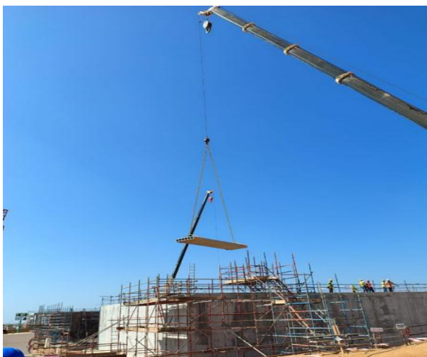
Fig 8: Typical erection of Hollow Core slab panel
