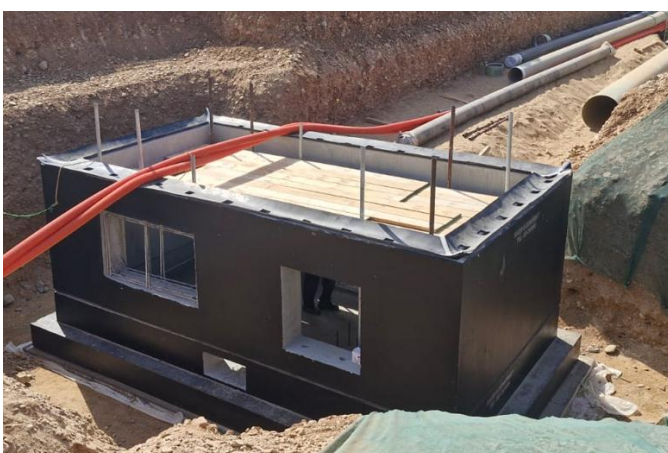
Fig.6: Raft & Wall segment aligned
