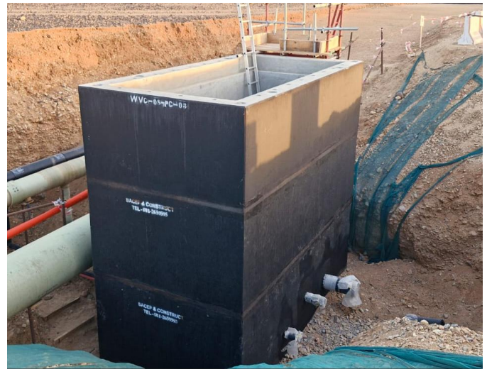
Fig.2: Precast segments erected & aligned
