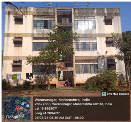
Fig -1: OLD RCC BUILDING ( G+2)
