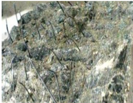
Figure 4.11 Failure of PFRC slab
