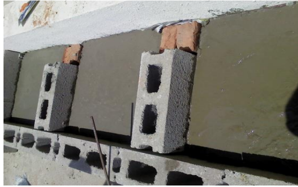
Figure 4.10 Laying of slabs
