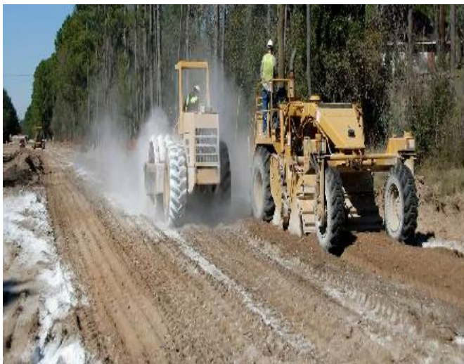
Figure-1: Soil Stabilization
