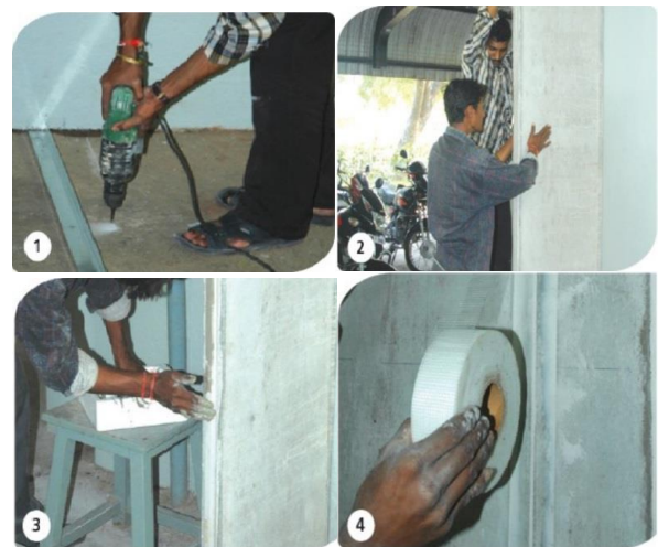
Fig. 5 Panel Installation Steps
