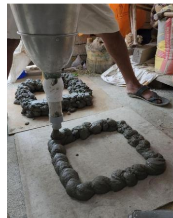
Fig -39: Extrusion progress
