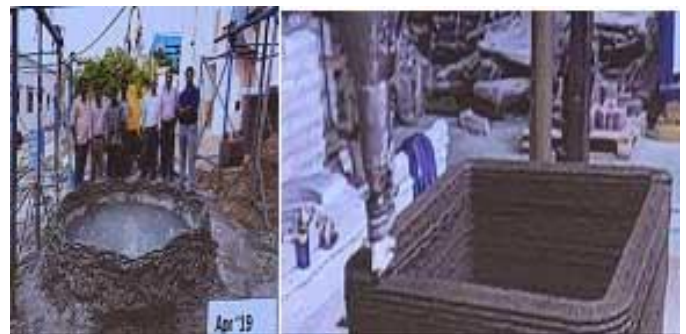
Fig -7: L & T has hand printed first water tank of capacity 2KL at Kanchi in year 2019 & First Trial with COBOD printer in year 2022
