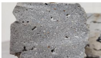
Fig -30: Enlarged view of core sample cross section: Strong and hard surface texture found. No serious issues with inter layer bonding.
