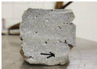
Fig -29: Core Samples cross section examination. No serious cold joints, shrinkage cracks or voids found
