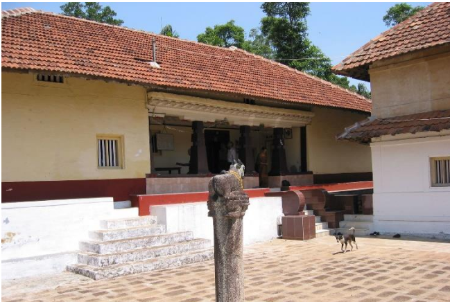
Fig -3: The Balladchanda Ainmane- Typical features of tapering columns in the Kayyale, the wooden Kaimara, Small windows, and steeply sloping roofs can be observed. The Kal Boti in the yard is also seen. [8]
