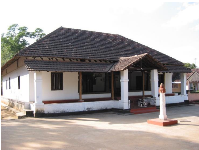
Fig -4: The Mukkatira Ainmane, built around 1870s, The front Veranda is an addition made in the 1910s. [9]
