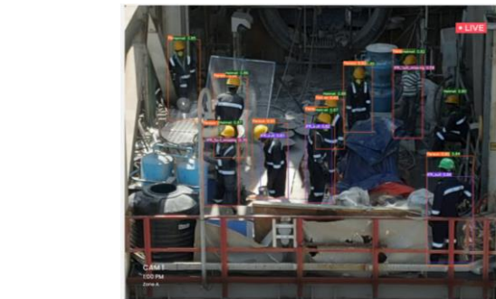
Fig -4: Real-time Detection of anomalies PPE kit (Helmet, IFR suit, Gloves, Shoes) and Mask.
