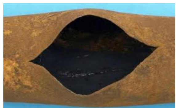
Fig:2 Short Term Overheating of Boiler waterwall Tube due to overheating.
