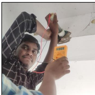
Fig.5 Half-Cell Potential difference test on RC beam
