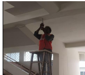
Fig.3 Rebound hammer test on RC beam
