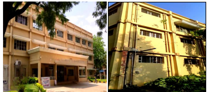
Fig. 1 General View of the Building
