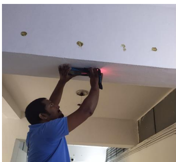
Fig.6 Profometer studies on RC beam
