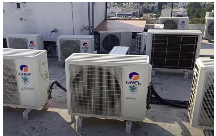
Fig:2 A residential terrace loaded with AC units
